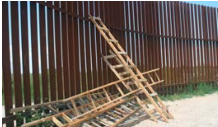
LADDERS ACCUMULATE ALONG A BOLLARD BORDER WALL IN TEXAS. PHOTO: SCOTT NICOL
